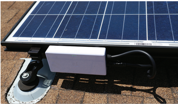
Solar Gateway Installed
