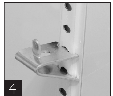
4 Shelf clip installation complete
