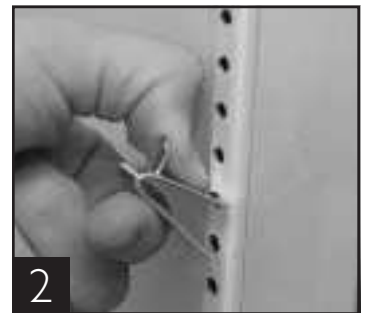
2 Installing bottom of the shelf clip
