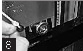
8 Door roller bracket with nylon cord.
