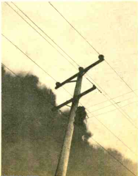
Size of insulators identify voltages: Three on top carry 34,500-v conductors. Below them are 7200-v lines. Bare wires extending to right are 110/220-v secondary wires running into home.
