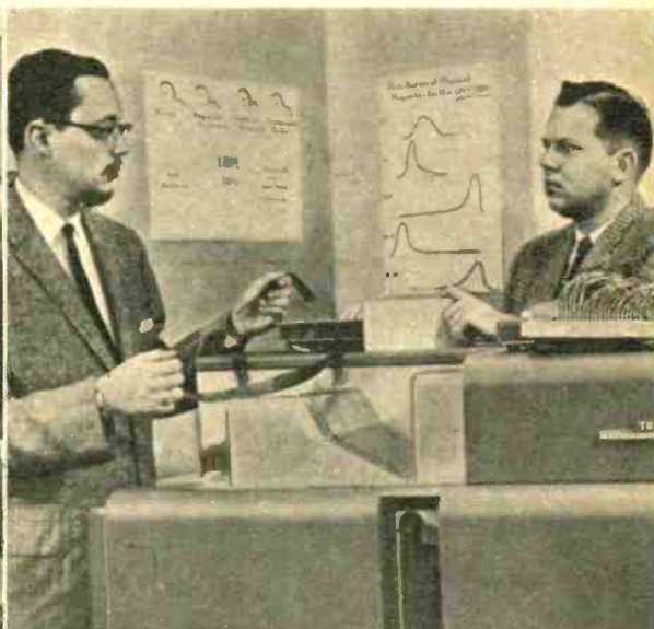
Data on punch cards held by R. A. Carpenter, right, has to be translated and prepared on magnetic tape for big Vanguard computer.
