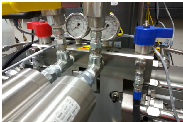
FIG. 27: HFR Manifold Valves in the Manual Circulation Positions
