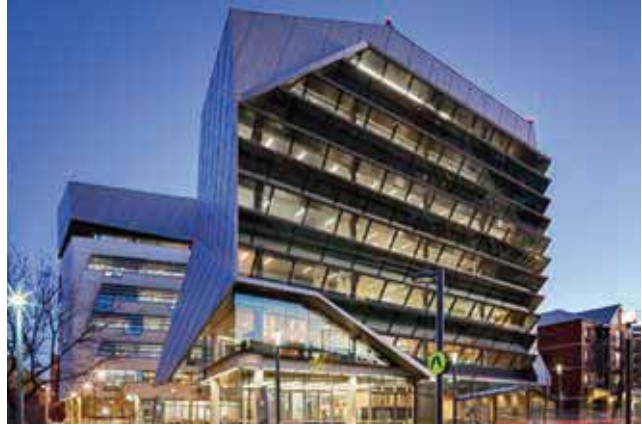
University of South Australia - Australia
