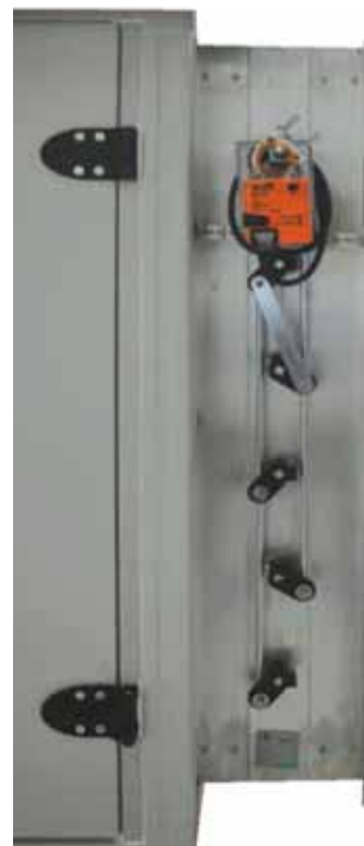
Damper motor inside and outside of the unit
