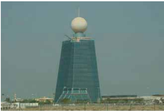
Etisalat Data Center, Fujairah - UAE
