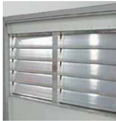
Parallel blade damper inside the air handling unit
