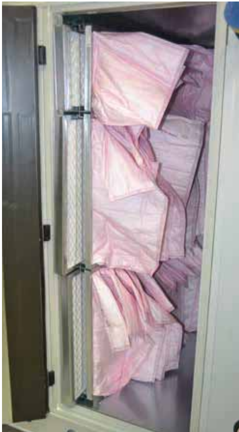
Side withdrawable combined filter (panel + bag)
