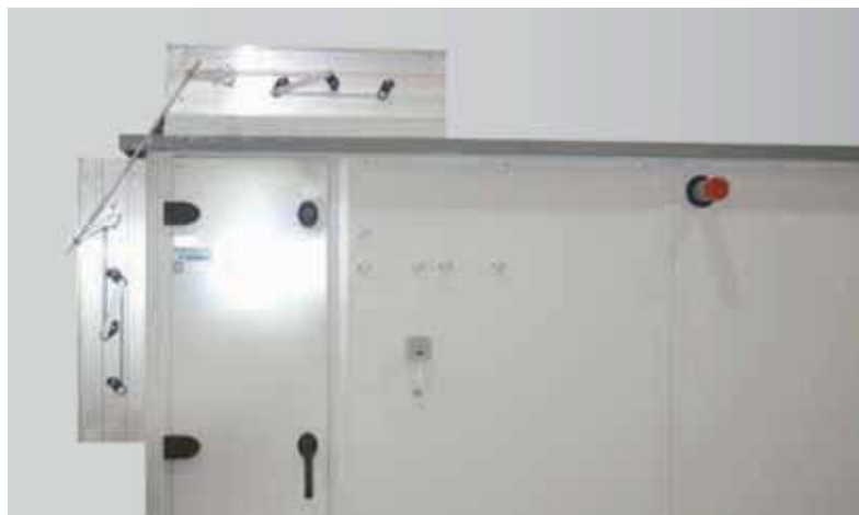
Internal or external damper actuator
