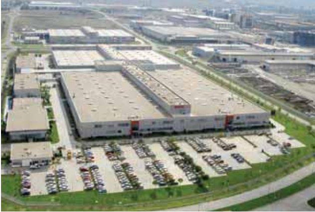
Boshch Diesel Injector Production Facilities - Bursa
