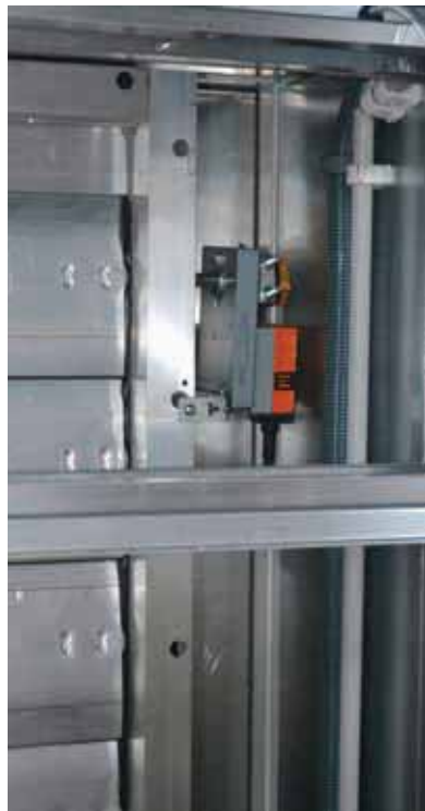
Internal or external damper actuator
