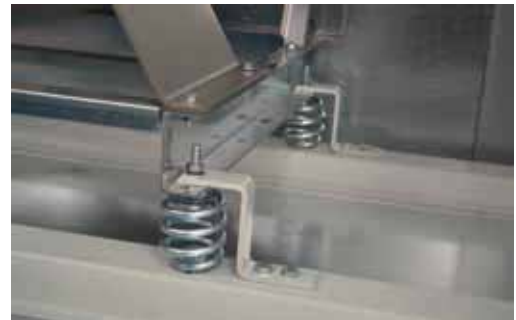
Spring anti vibration mounts
