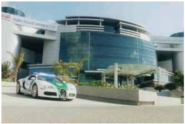
Siemens Headquarters, Dubai - UAE
