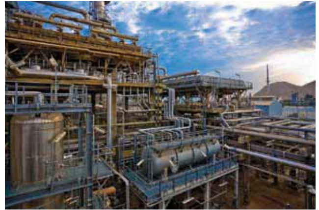
Sohar Refinery - Oman
