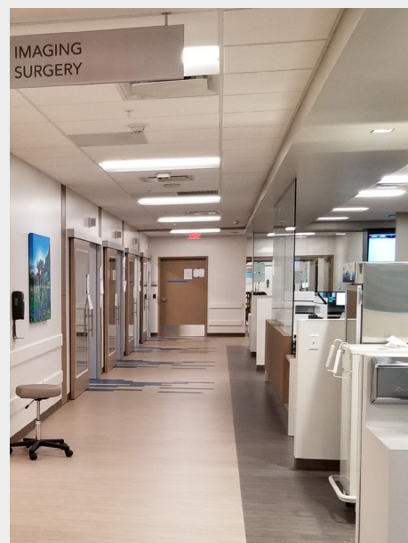
AD Systems™ sliding doors were used for exam rooms to save space and reduce noise.
