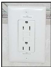
Figure 7-7. GFCI Receptacle
