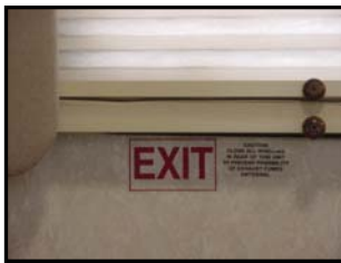
Figure 13-2. Emergency Exit Window
