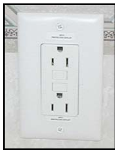
Figure 7-5. Typical AC Receptacle
