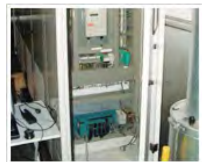
STARDOM controller installed in the site cabinet
