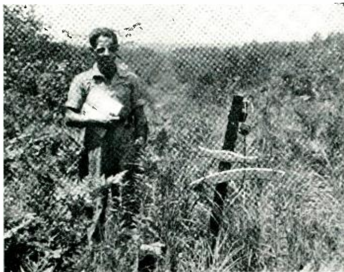
Fig. 4—Cable depth indicator in use. Notes were kept for the plow operators
