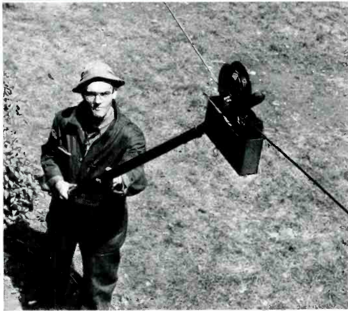
Fig. 2—Albert J. Oppel, repairman in the Newark Suburban District of the New Jersey Bell Telephone Company, uses a drop-wire painter that is attached to a tree pruner handle to permit weather-proofing from the ground
