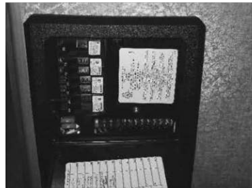
Figure 9-9: Main 120 VAC Load Center
