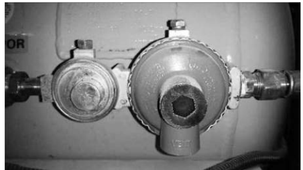
Figure 2-4 LP Gas Regulator
