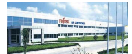
Fujitsu General (Shanghai) Co., Ltd. (China)
