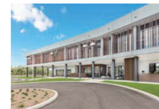
Fujitsu General (Aust.) Pty Ltd. (Australia)
