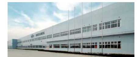
Fujitsu General Central Air-conditioner (Wuxi) Co., Ltd. (China)
