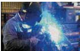
All welds completed prior to PermaGlas Ultra Coat.
