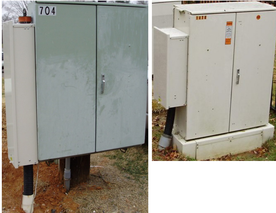
Figure 1: Completed Add-On 400 Pr. Annex NetReach™ Expander® Cabinet Installation (left-hand installation shown for left: 1x8 Expander® cabinet and right: 2x4 Expander® cabinet).
