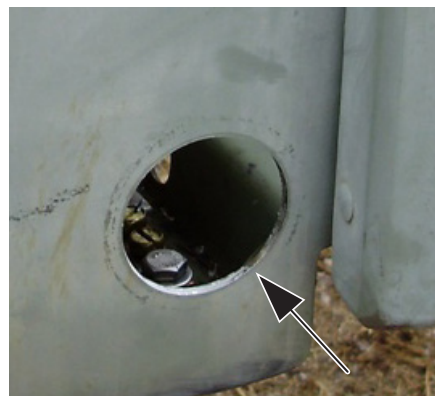
Figure 5: Marked and drilled 1-3/4" hole at the lower left-hand side of the host Cross-Connect cabinet.
