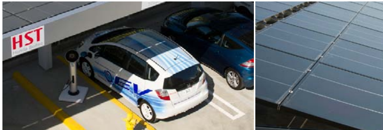
Honda CIGS thin-film solar cells installed on the roof and carport of Honda Performance Development in Santa Clarita, California.
