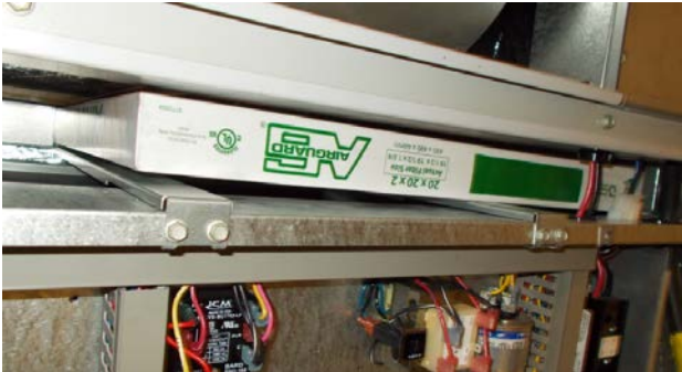
FIGURE 10 Install Left 2" Filter
