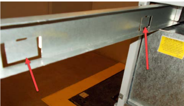
FIGURE 5 Bend Filter Tabs Down
