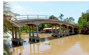
A bridge on the school commuting route
