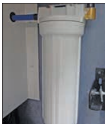
Figure 13-8: Water filter
