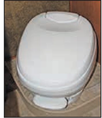
Figure 13-10: Toilet pedal flush lever
