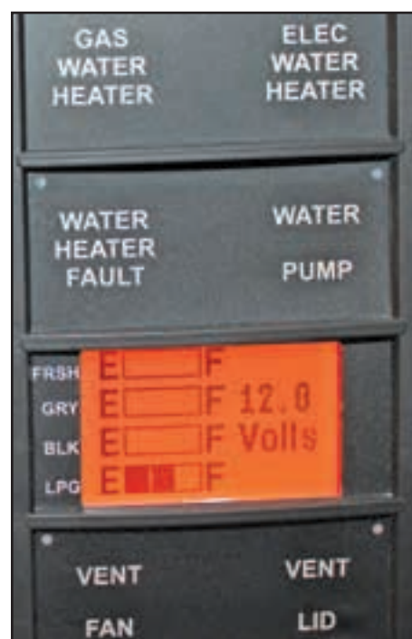
Figure 5-7: Water heater switches
