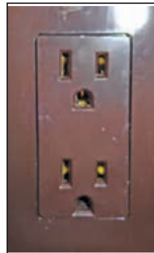
Figure 9-2: 120 VAC receptacle
