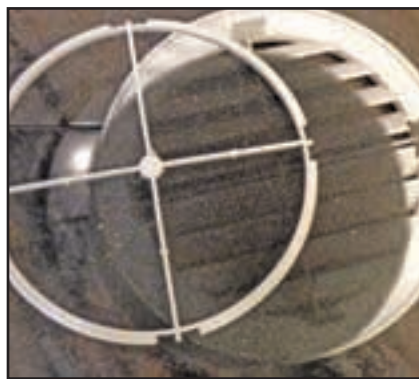
Figure 3-3: Round vent filter
