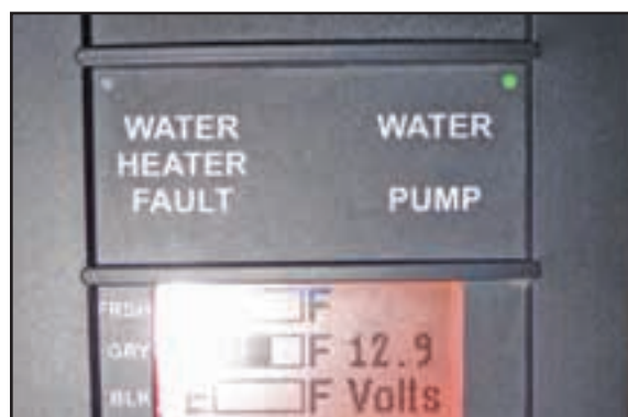
Figure 13-5: Water pump switch
