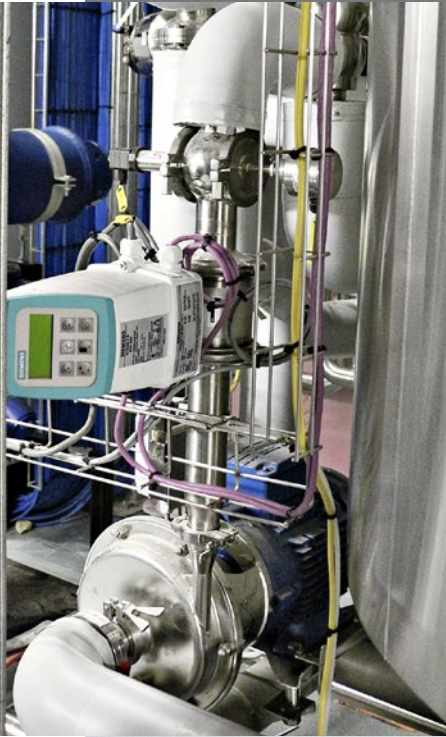
A strong team: Sitrans F M MAG 6000 with Sitrans P compact and Sitrans TS300 for precise measurements of flow, pressure, and temperature ...
