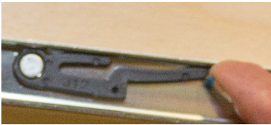
Typical left-hand (LH) side plastic kitchen drawer release clip, shown above.
