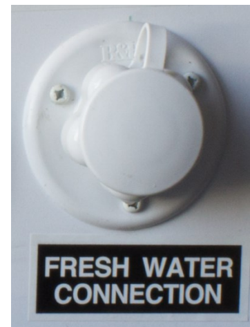
Typical city water inlet
