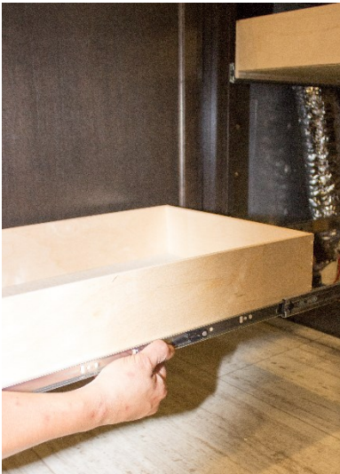
Typical kitchen drawer removal, shown above.
