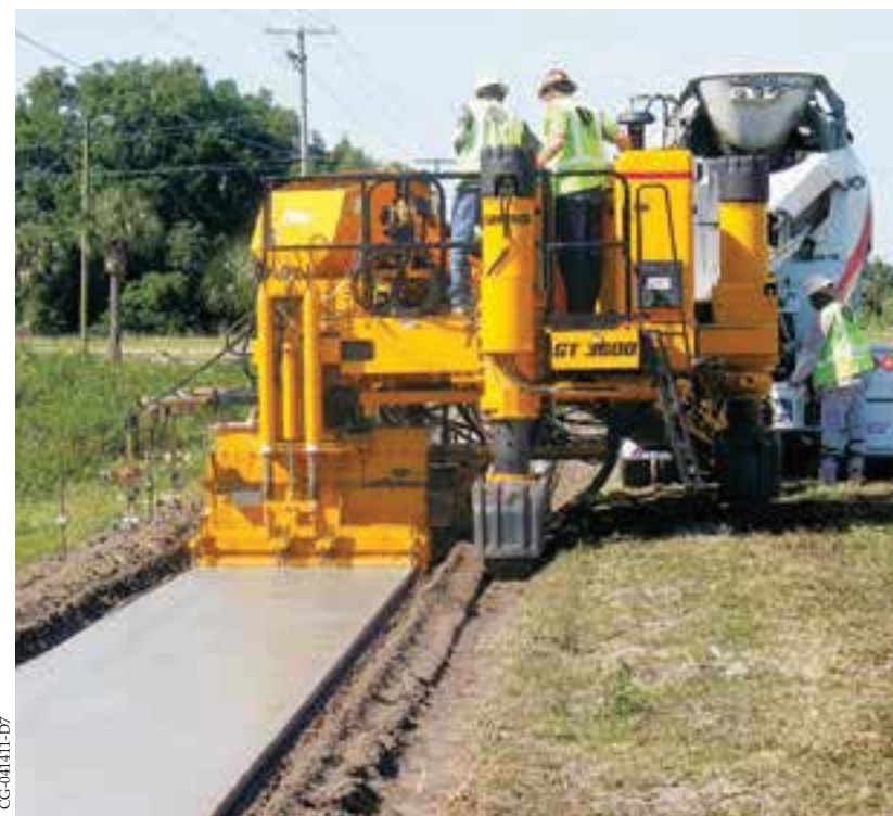
Minimum-clearance, versatility, and high production are achieved with the GT-3600 as it slipforms this five foot (1.5 m) wide sidewalk.
