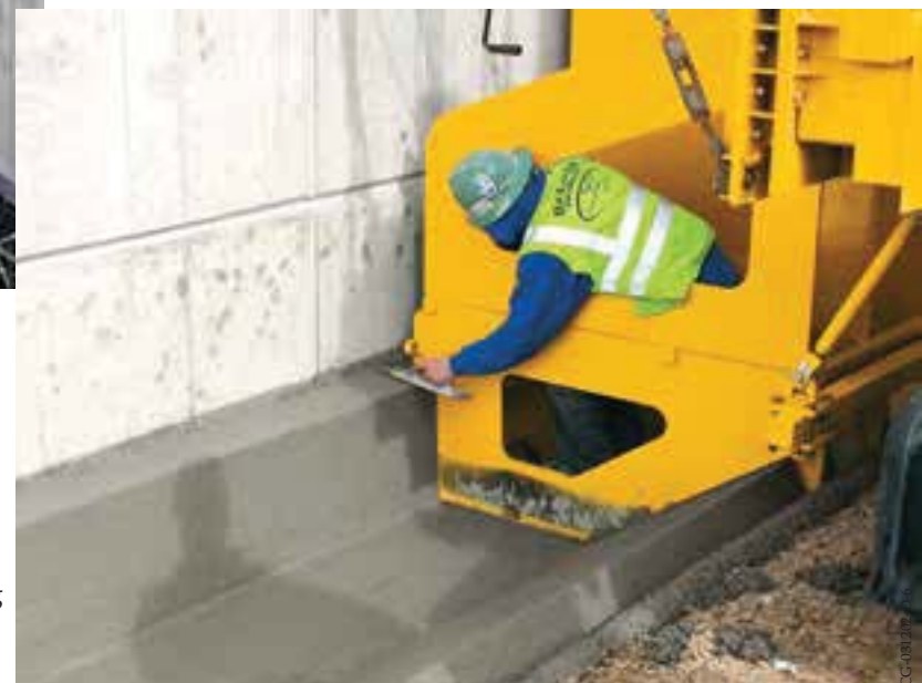
A crew member works behind the GT-3600 putting the finishing touches on a drainage channel.
