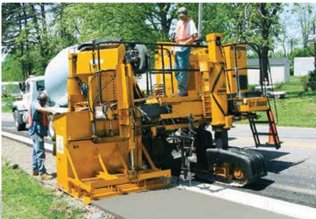
The GT-3600 with All-Track Positioning (ATP) provides easy setup for slipforming sidewalks. Steering and grade are referenced off the existing curb.
