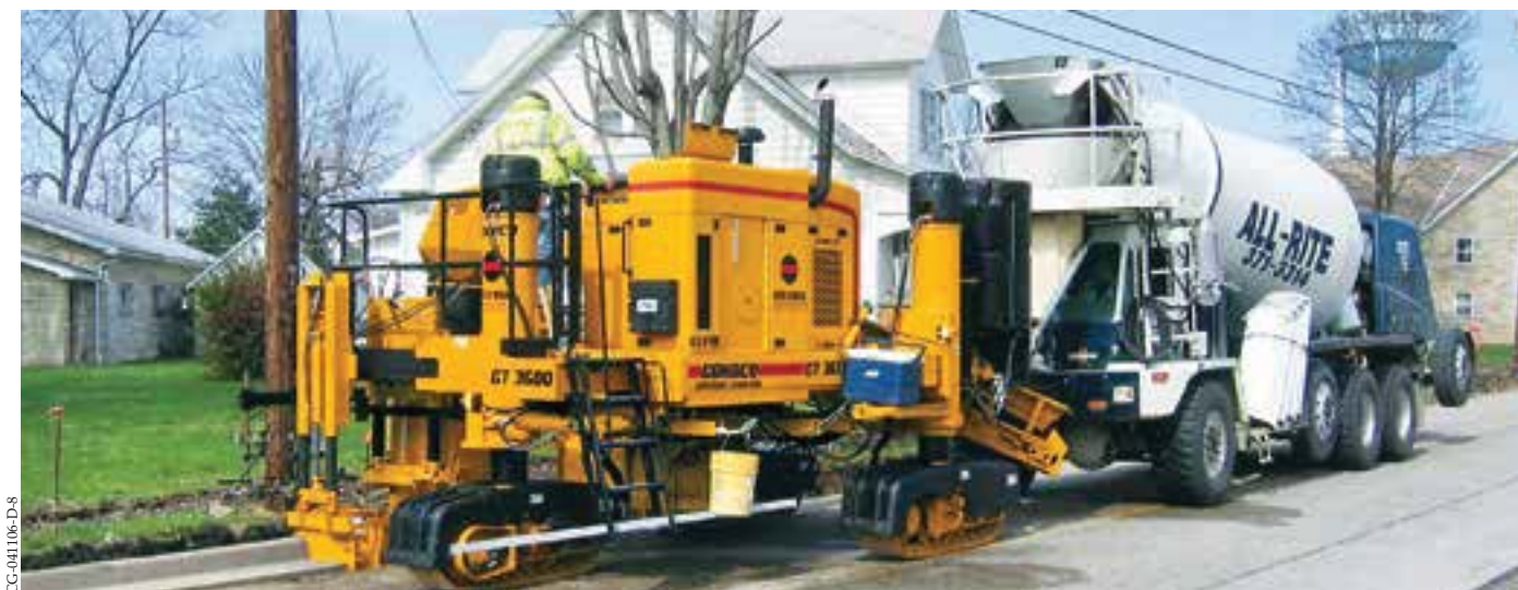
This GT-3600 slipforms curb and gutter below grade on a rehabilitation project. Using the telescoping mold and hold-down, the GT-3600 is able to achieve minimum-clearance as it passes a residential telephone pole.
