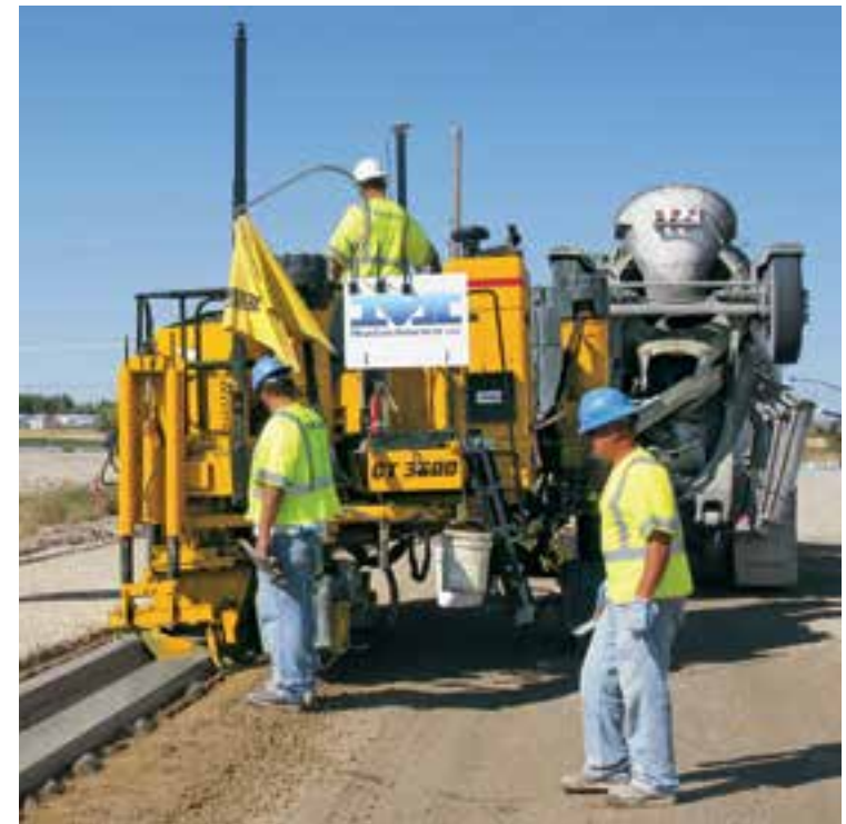
Stringless curb and gutter is slipformed on a new parking lot project with 3D stringless controls.
