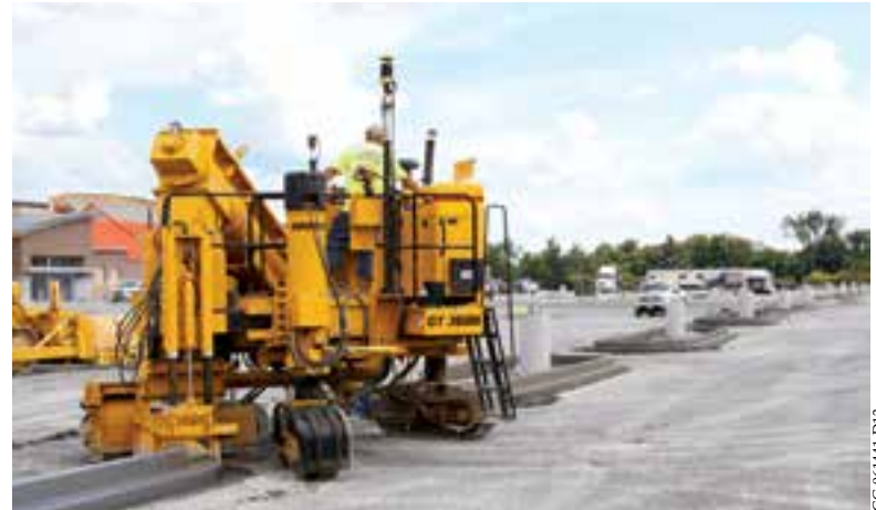
The GT-3600 with 3D machine guidance slipformed radii as tight as 2.5 feet (0.8 m) on this parking lot project in Tennessee.
