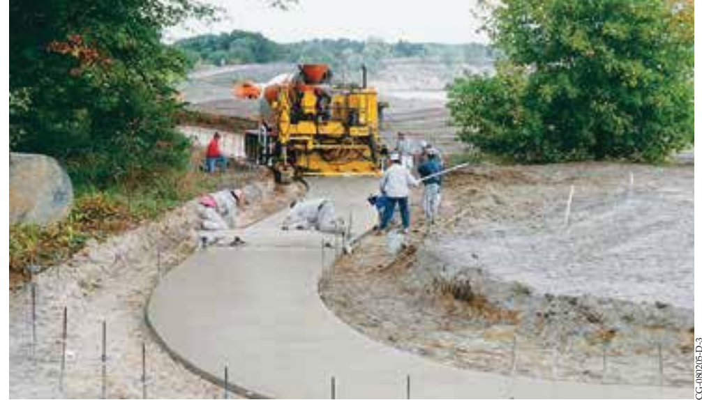
The GT-3600 slipforms 18 holes of continuous golf cart path. This golf cart path is eight feet (2.4 m) wide, four inches (102 mm) thick, and 30,200 feet (9205 m) in length. The total amount of slipformed concrete required was 3020 cubic yards (2309 m 3 ).
