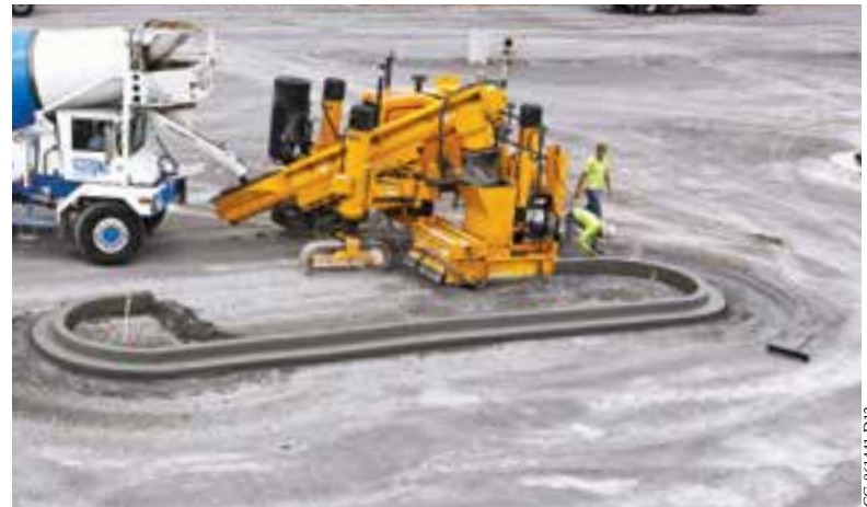
The GT-3600's All-Track Steering, combined with the 3D system's steering algorithms, allow smooth entrances and exits and tighter cornering for tight radii work.
