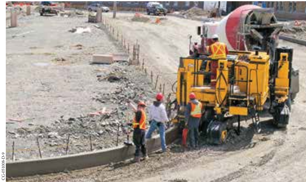
This GT-3600 slipforms a 16 inch (406 mm) curb in Canada.
