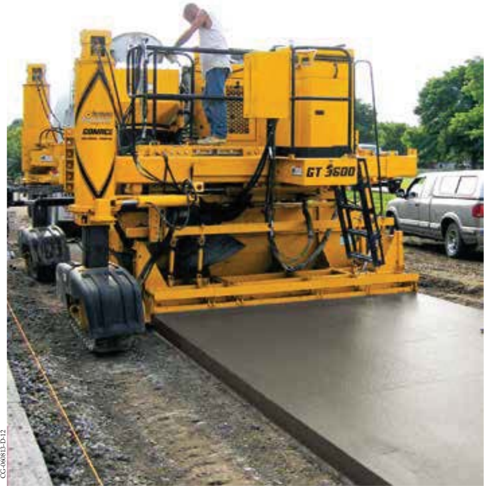
The GT-3600 slipforms a 10 foot (3 m) wide sidewalk with a center-mounted mold.
