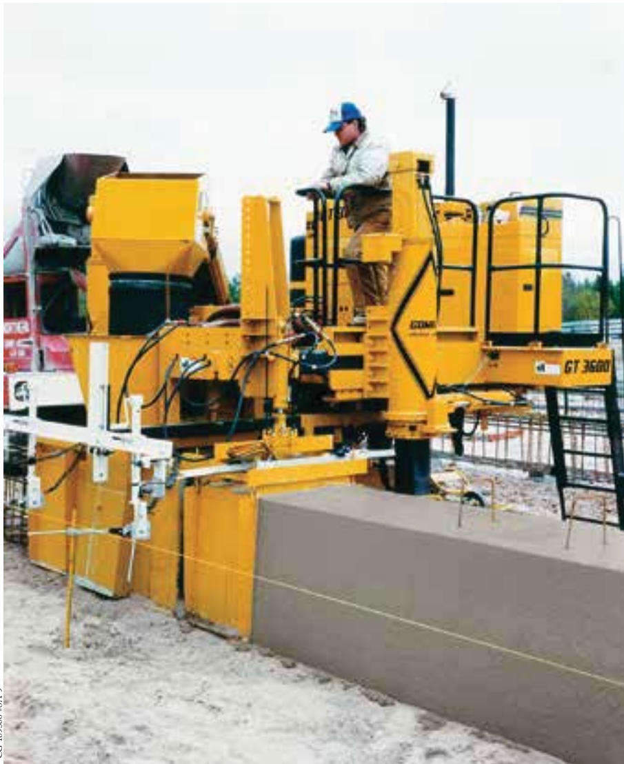
A GOMACO GT-3600 slipforms the foundation for an ice skating rink in Michigan.
