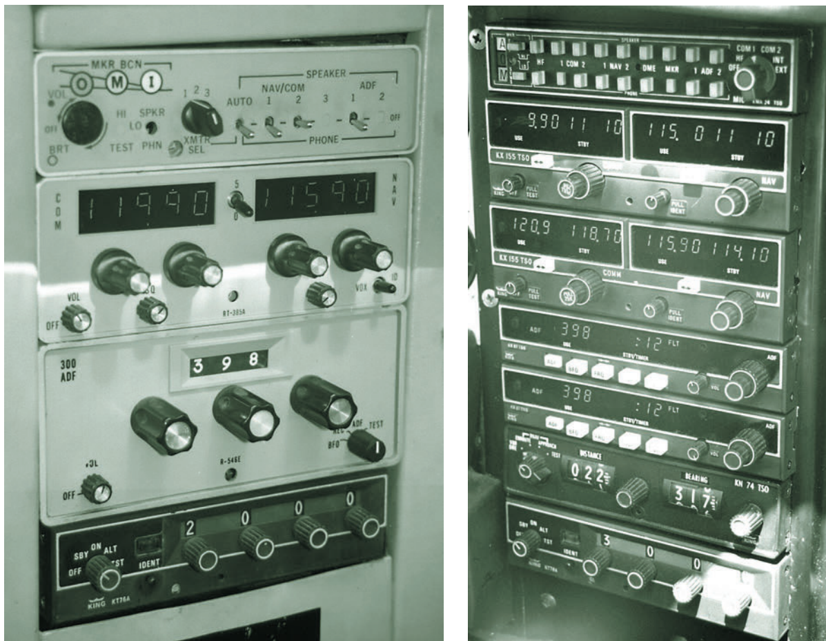
Figure 1-20 Radio control panels.
