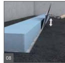
Apply thinset mortar to support the profile at desired height.
