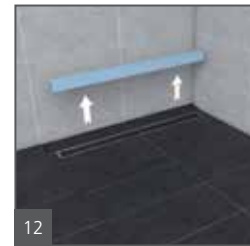
Remove the foam block spacer.
