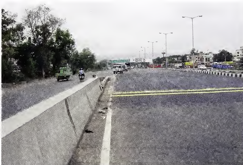
Fig. 5.32 Improperly Designed Merging Point of Expressway and National Highway
