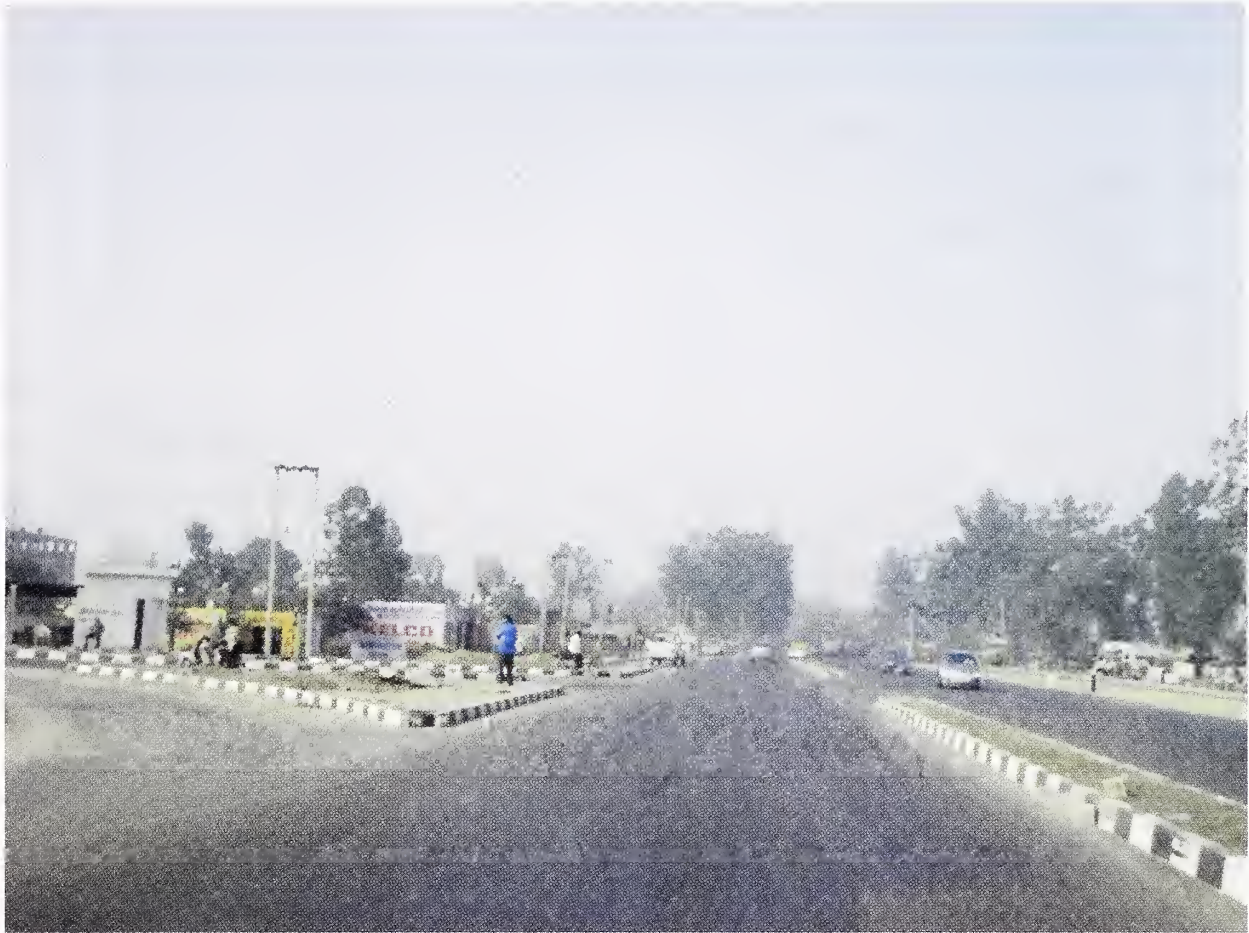
Fig. 5.16 Large Channelising Island
