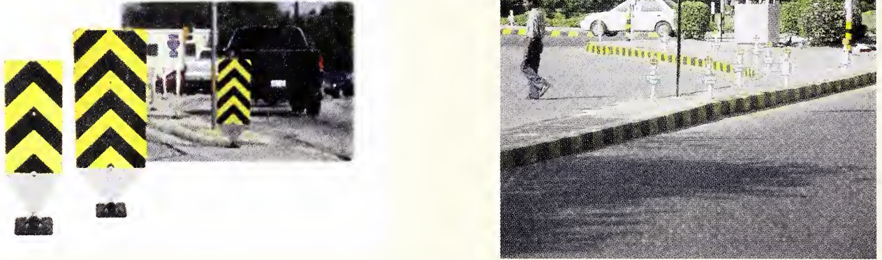
Fig. 5.30 Delineators and Chevron Signs
