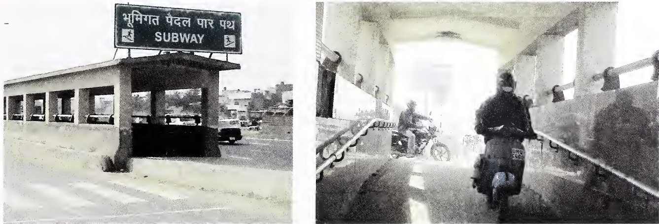
Fig. 6.3 Poor Quality Design of Subway at Access Controlled Highway
