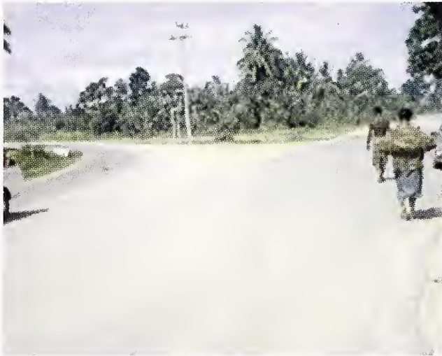
Uncontrolled Y-Junction with no markings, priority or traffic islands causes conflicts and uncertainty between merging and opposing traffic
