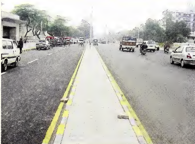
Well Maintained Median Width with Proper Median Markings
