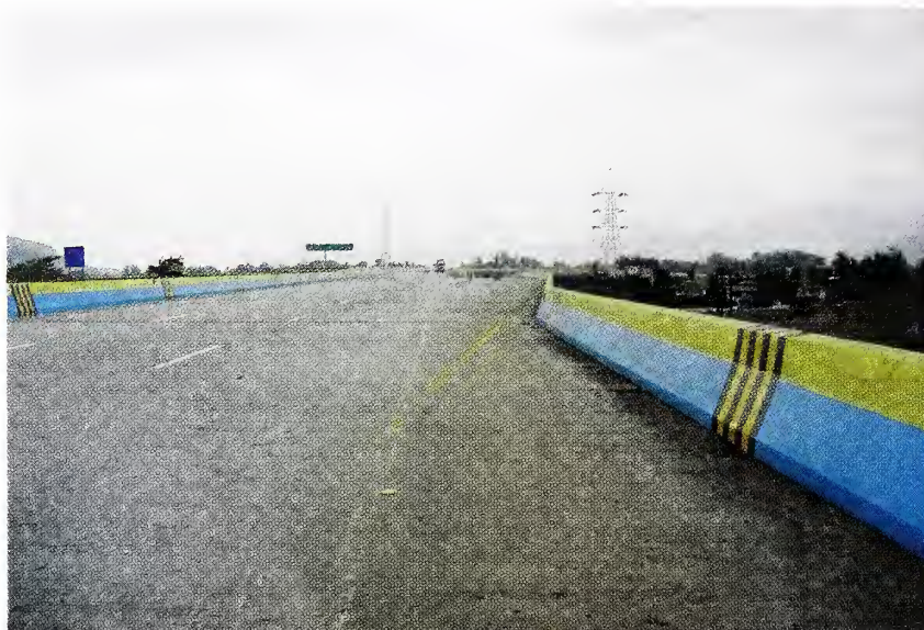
Fig. 5.31 Merging Area Inadequately Designed and Provided with Proper Signs
