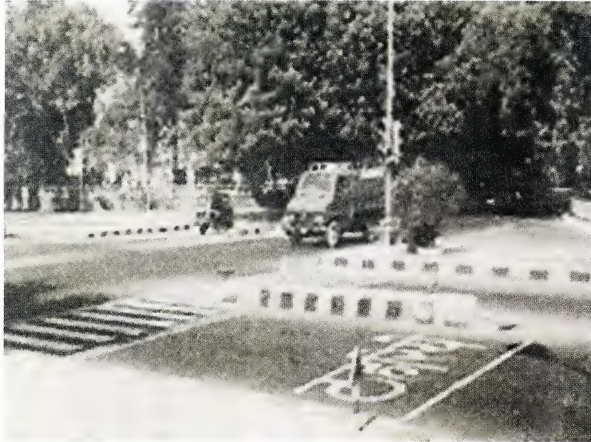
Fig. 5.14 Well Marked Junction with Proper Road Markings to Assist Drivers and Enhance Safety
