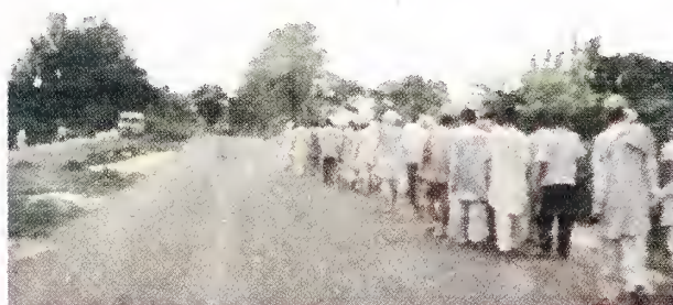
Lack of rural footways forcing pedestrians to walk on the carriageway in India
