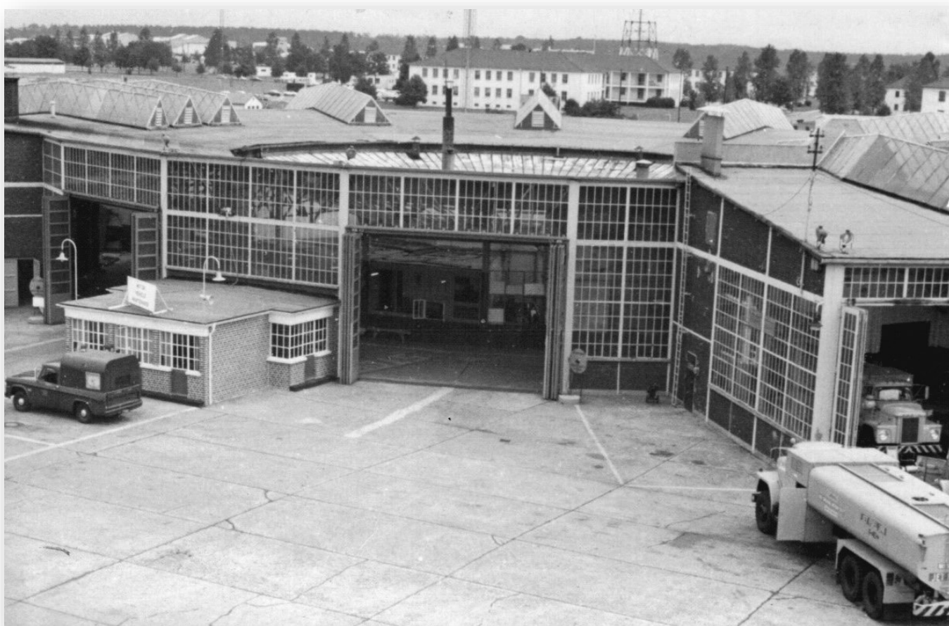
VEHICLE MAINTENANCE SHOP KNOWN AS "THE ROUND HOUSE" RHEIN-MAIN AIR BASE, GERMANY — CIRCA 1980. THE WHITE SIGN ON TOP OF THE RECEPTION CENTER (QC) SAYS "MOTOR VEHICLE MAINTENANCE"
