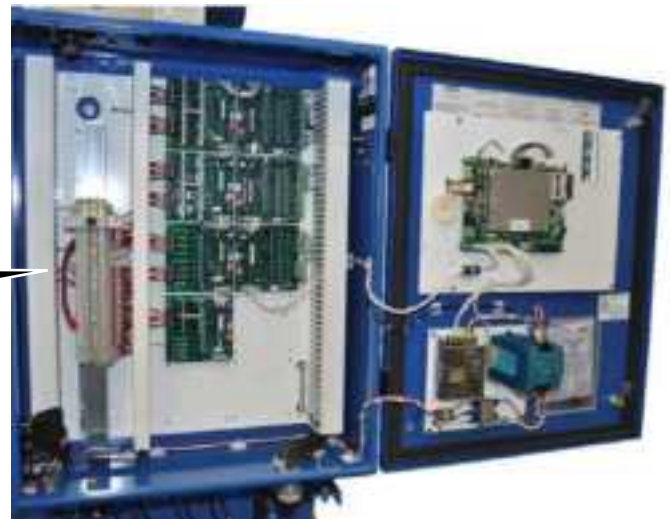
Figure 4-5. Wire Connections for Capacity and Volume Actuators
