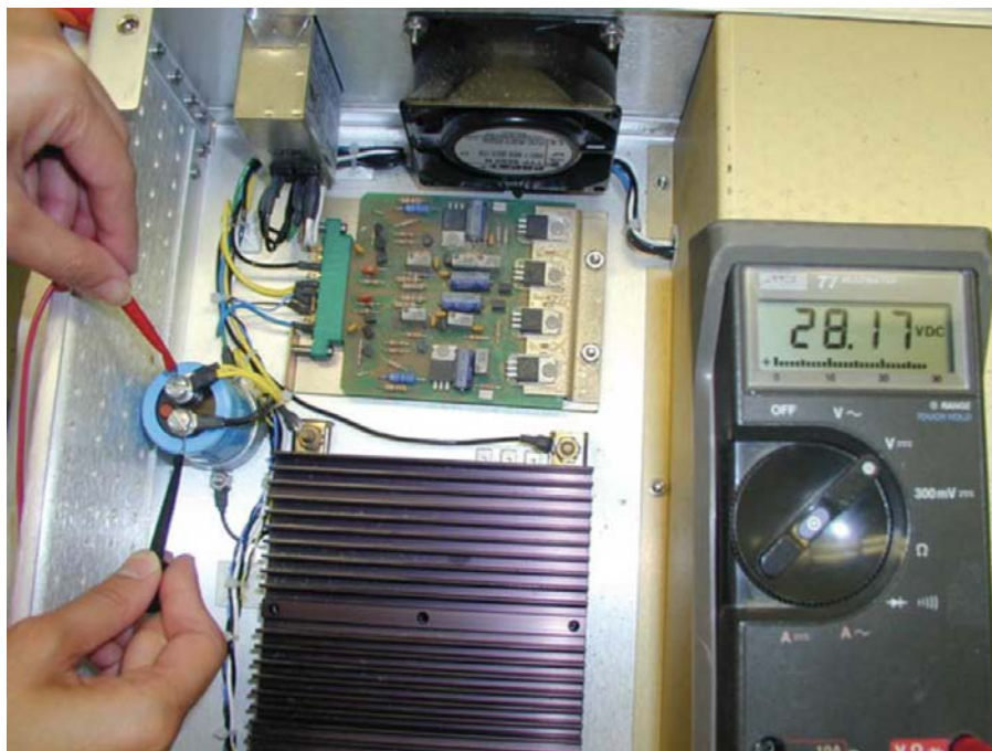
28V DC power supply measurement.
