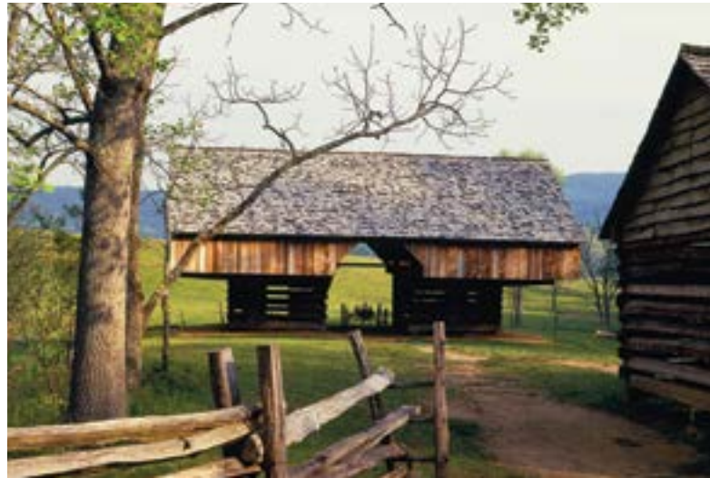
The cantilevered barn is unique to the Southern Appalachians, characterized by a large overhanging second story. This architectural style was used frequently in Blount and Sevier counties.
