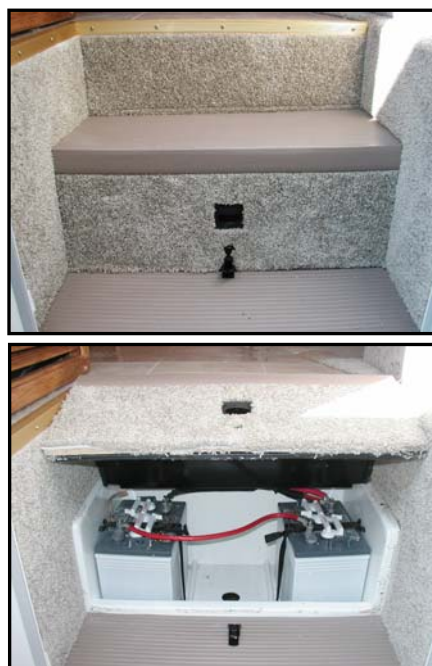
Figure 7-3. Stairwell (Top) and Battery Storage Underneath (Bottom)
