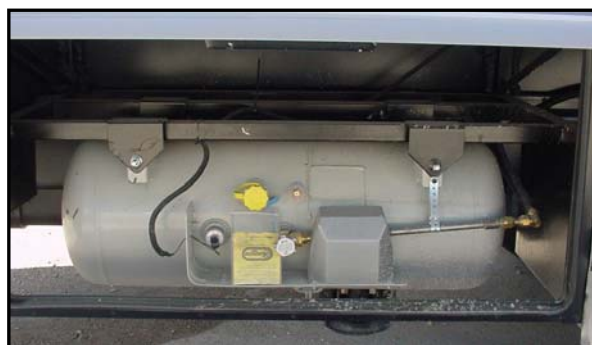
Figure 2-4. Liquid Propane Tank
