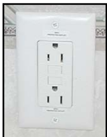
Figure 7-7. GFCI Receptacle
