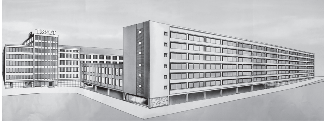
1965 construction project, Tissot's North Tower.
