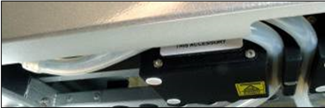
Hoses visible in the gap between the rear cover and the pinch valve.
