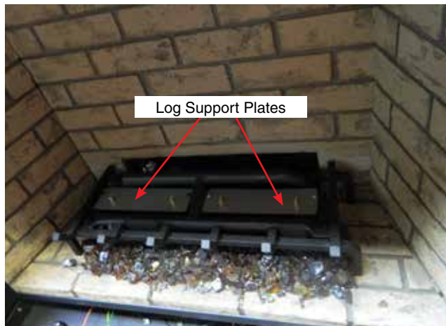
Diagram 6—Log support plates installed
