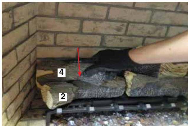
Diagram 10—Install Log 4
