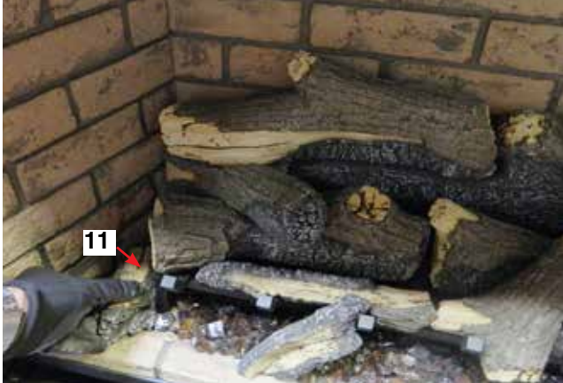
Diagram 17—Install Log 11
