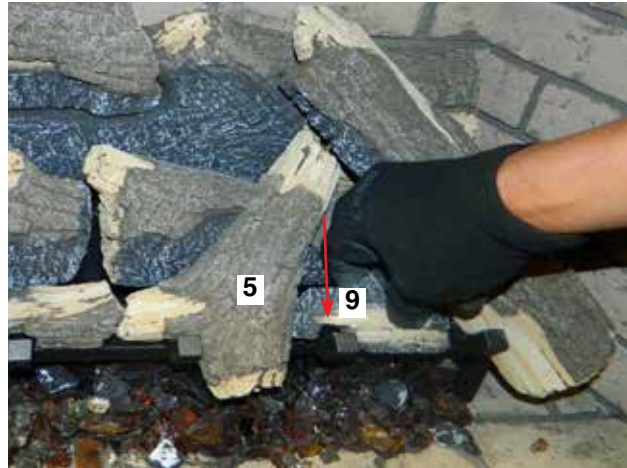
Diagram 15—Install Log 9
