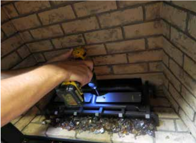
Diagram 5—Install Log support plates
