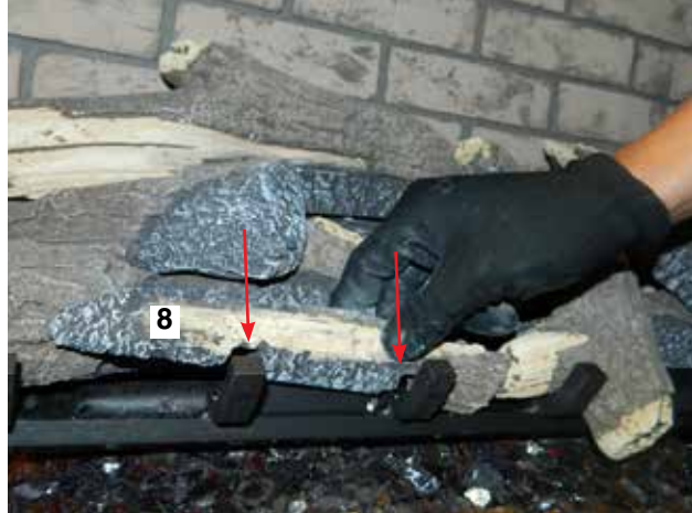
Diagram 14—Install Log 8
