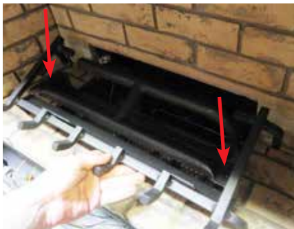
Diagram 1: Remove the left and right screws.
