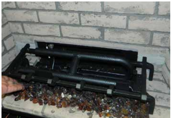
Diagram 4—Install Vermiculite + Lava
