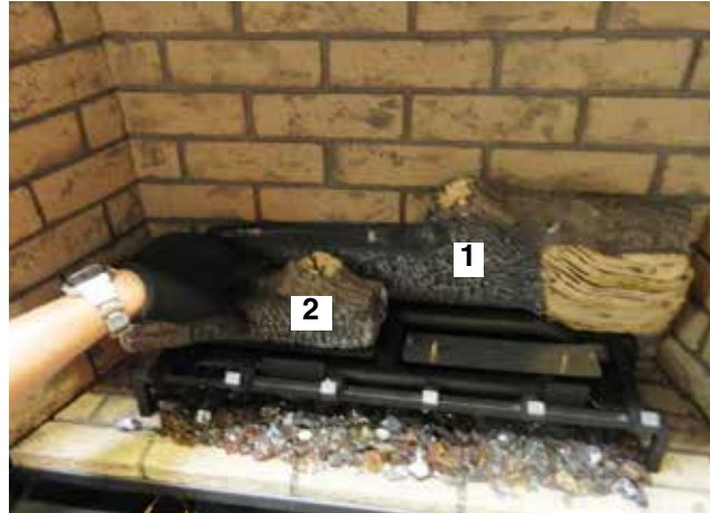
Diagram 8—Install Log 2
