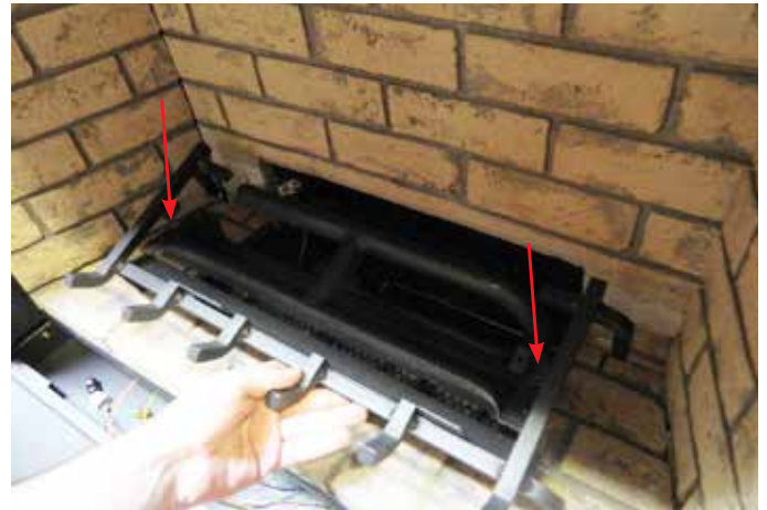
Diagram 2—Log Grate Install
