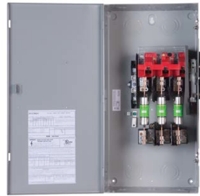
Figure 2. Safety switch with door open
