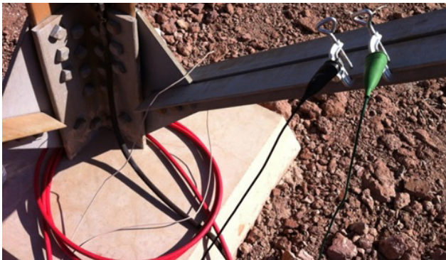
Output leads installed on a tower leg
