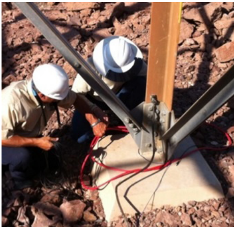
Installing the GroundFlex® probes (in this illustration, the probes are looped twice around the tower leg)
