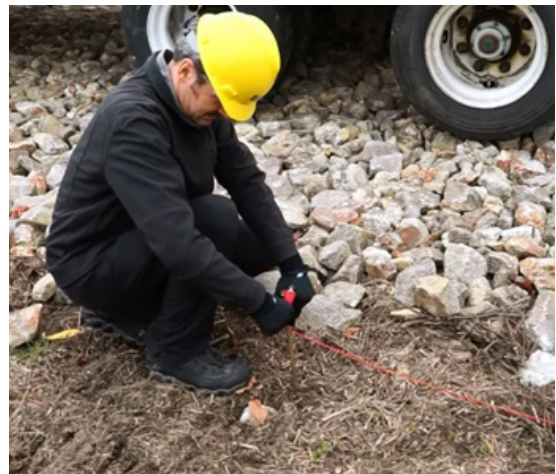
Installing an electrode
