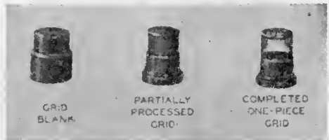
Fig. 8—Fabrication of one-piece grid.
