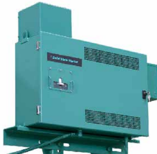
FIGURE 14 - UNIT MOUNTED LVSSS (ECONOMIZER)
