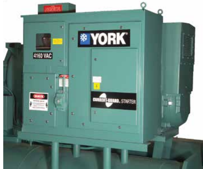
FIGURE 13 - UNIT MOUNTED MVSS
