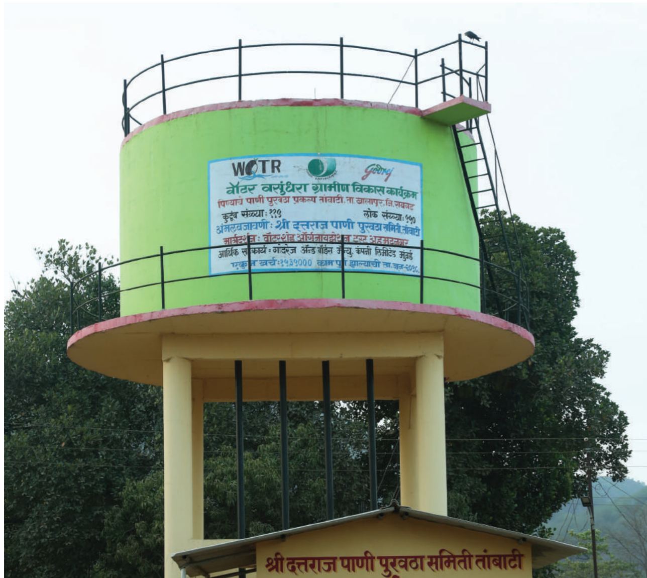
Varied capacity water tanks built at Khalapur village of Tambati & Vadval.
