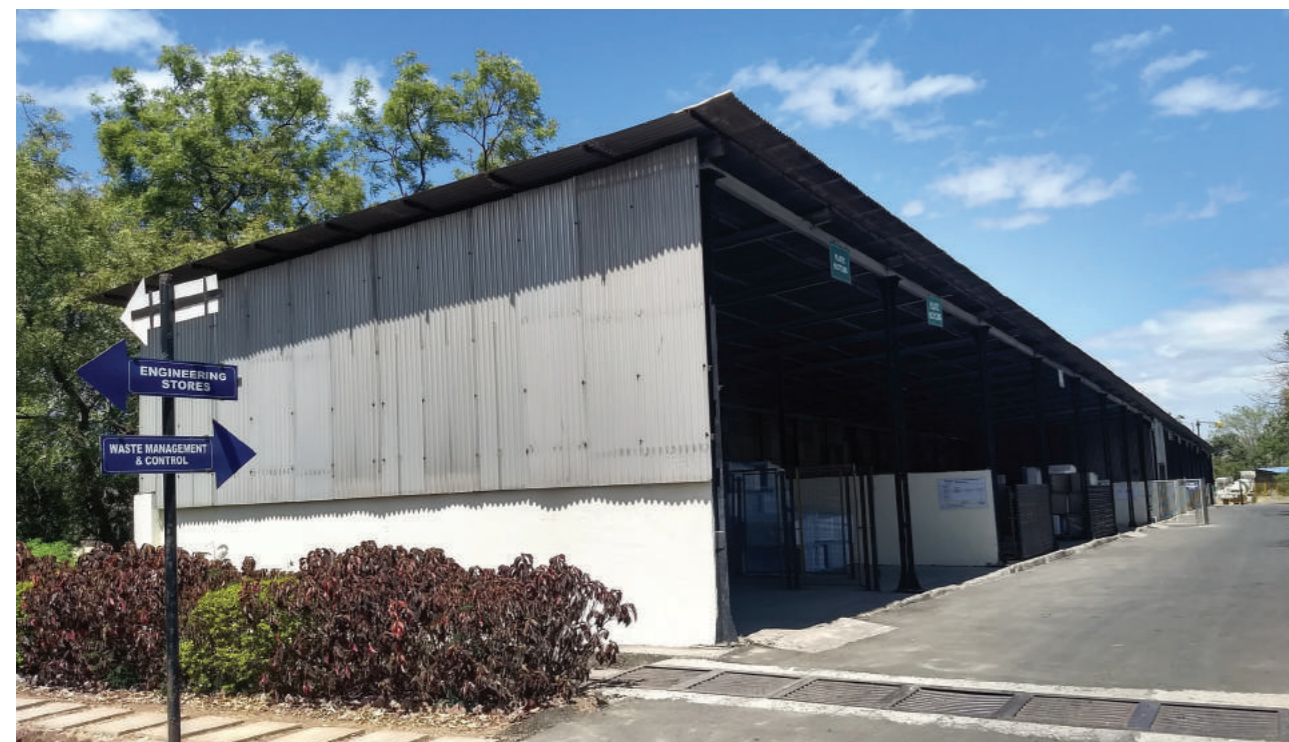
waste management yard at Godrej Appliances plant at Shirwal
