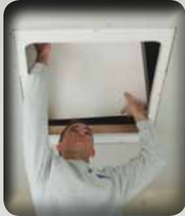
3 Install drywall and place access panel in opening.
