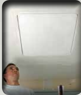
4 Tape and apply drywall compound.
