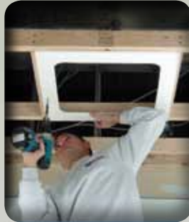
2 Mount Stealth surround with drywall screws.
