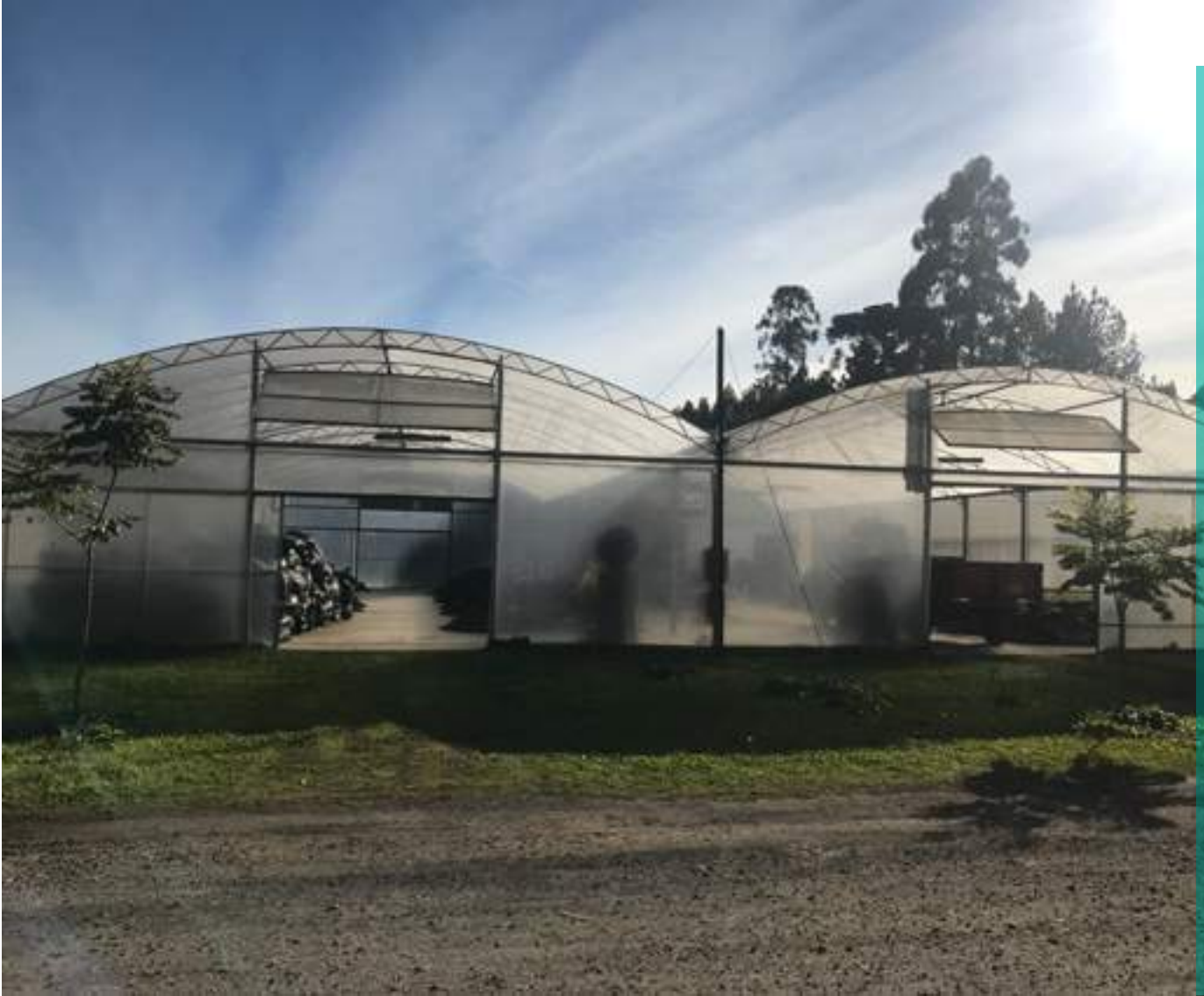
Composting processes – composting greenhouses
