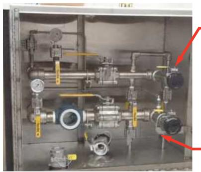
The fill box, pictured here, is a good place to connect the nitrogen bank and the recommend location for pulling vacuum. Use the hose provided and connect to the 1" vapor Epsilon fitting. The other hose end can be fitted with a connection for the nitrogen bank or vacuum pump.
