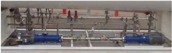
There are a lot of valves on the bottom of the tank to open, be sure to get them all. You can use the pressure gauges to monitor pressures. There should also be bleed points to relieve the pressure during the purge step(s).
