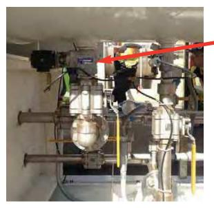
Some valves may be air operated and may even need a signal from a panel to open the valve. It is important to ensure all valves are in the open position.
