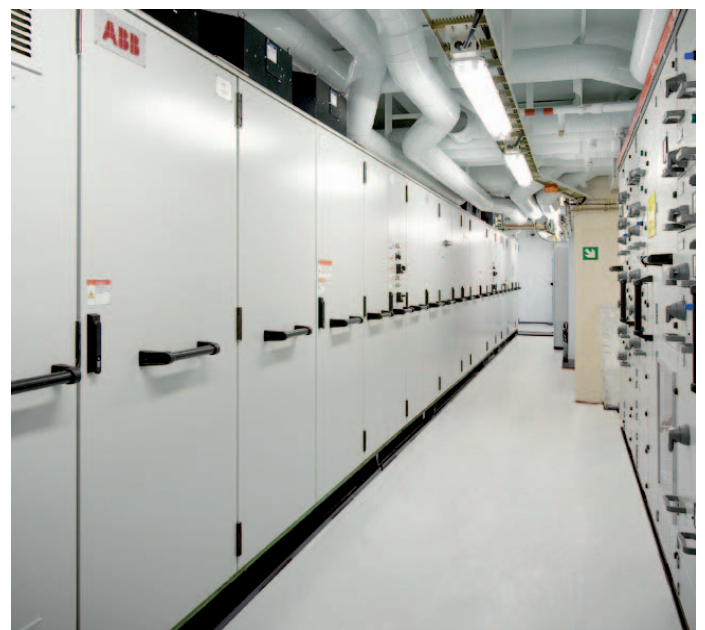
ACS 6000 variable speed drives controlling Azipod® propulsion motors
