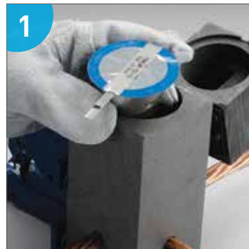
1 Insert ERICO CADWELD PLUS cup into mold (may require use of a cover/baffle)
