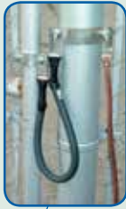
Fence and Gate Jumper Assemblies
