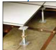
Signal Reference Grid (SRG)
