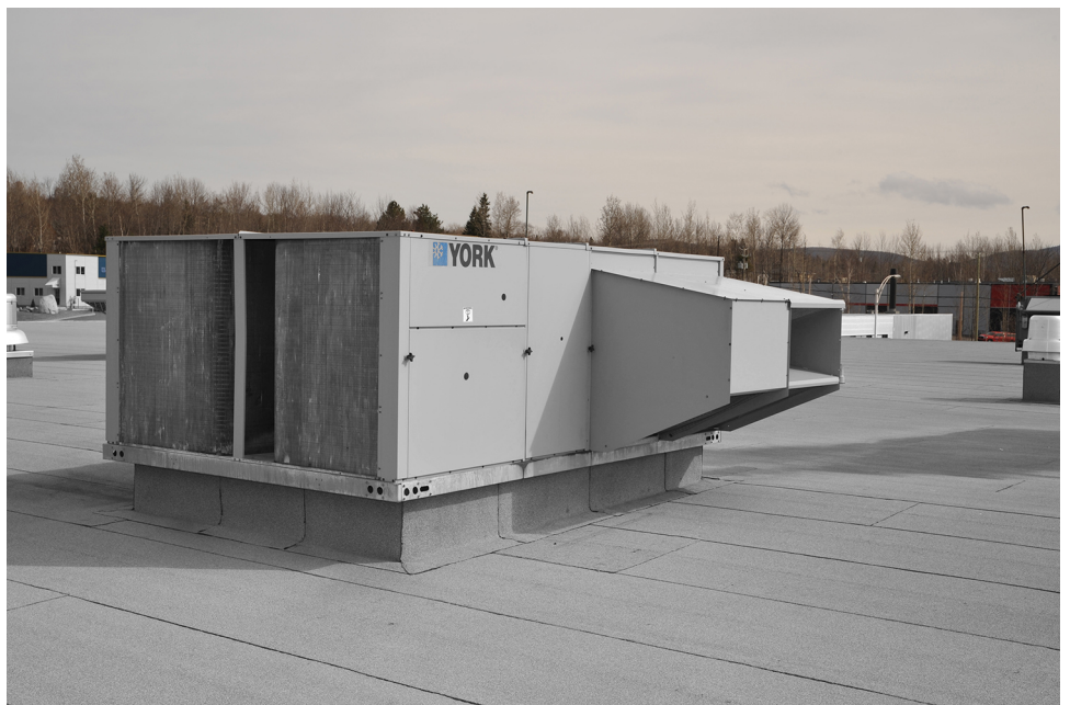
Figure 5. Typical air-handling unit.
