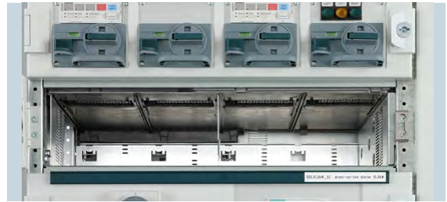
Fig. 4/15: Adapter plate for small withdrawable units
