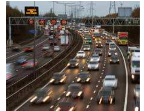
We provided preliminary and final design services for England's Smart Motorways.
