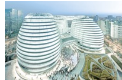
Galaxy Soho Office Building, Beijing (China)
