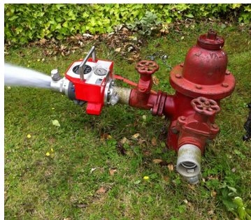
Fig. 1.3 Testing pillar fire hydrants on high pressure ring main
