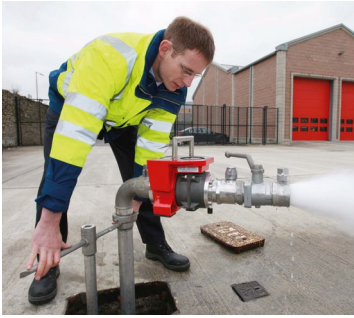
Fig. 1.2 Testing underground fire hydrants
