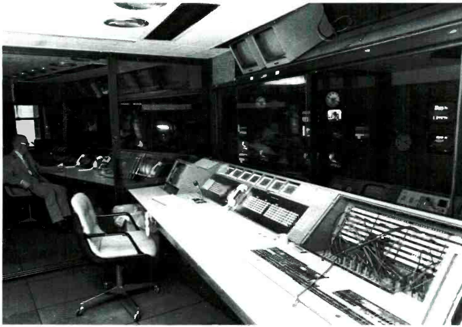
Fig. 1 — This photo of the Broadcast Operations Coordination (BOC) office shows what can be done to achieve a "built-in" custom look with standard telephone equipment. In addition to standard make-up hardware ("broker" phones and call directors), a patch bay (right) has been assembled with standard parts and centralized within the console area. All Telephone Company instruments within the Television Central complex (as well as selected peripheral instruments in other operating areas) may be interconnected from this patch bay. Thus, allowance has been made for the expansion and flexibility required under heavy traffic conditions.
