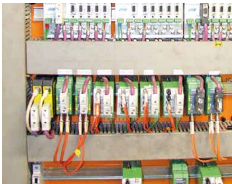
If the PB-XEPI is configured as a listener, the diagnose-tool is able to monitor the whole network without an own Profibus address
