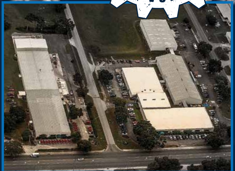
HALE's 140,000 ft 2 (13,000 m 2 ) Manufacturing Facility in Ocala, Florida
